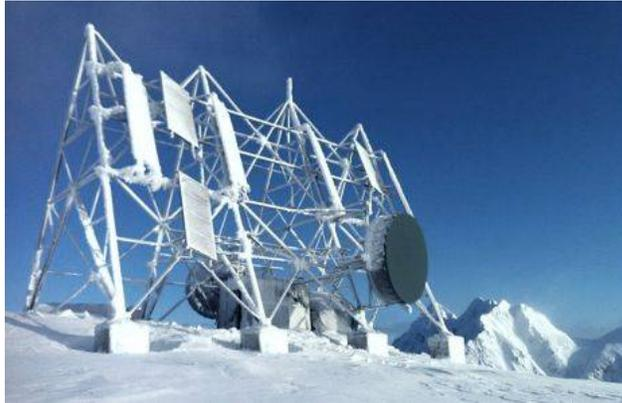
Fig. 1: Off-grid Microwave Radio Station with SOFC-PV Hybrid Configuration in Alaska – Sunfire-Remote 400 installed 2019
